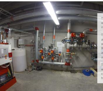
The fire protection supplied by Incendium covers two bunkers and one  $13.000 \text{ m}^2$  warehouse with plastic baled waste. These areas are protected with foam monitors and infrared cameras (IR).
